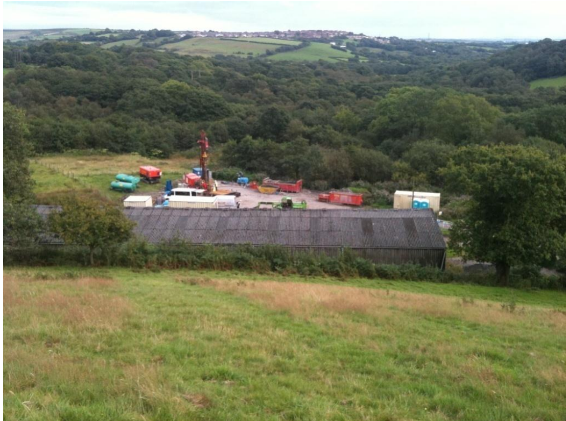
Figure 4: Drilling of Llangeinor 2 borehole
